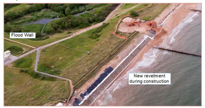
customer service line 03708 506 506 incident hotline 0800 80 70 60 floodline 0845 988 1188 Over 100 'Dycel mattress' panels have now been installed, forming a flexible mat of hollow concrete blocks that will extend the existing defence in this location. Recent efforts have been focused on completing the new access steps beyond groyne 3, which will be open in time for the school summer holidays on the 24<sup>th</sup> July.
